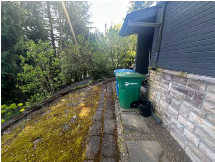
Eastern portion of residence
